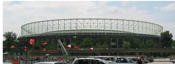
Ernst-Happel-Stadion, Vienna, built in 1929-1931, Renovated 1986
